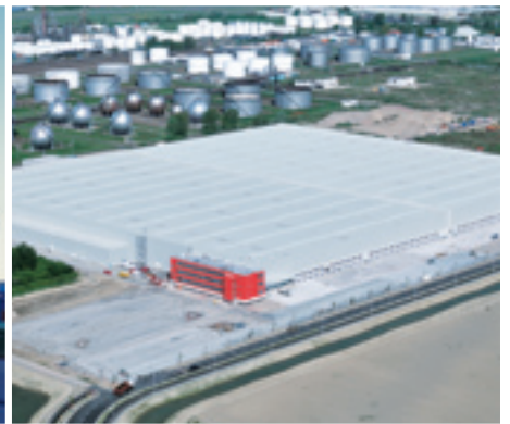
Pneuhaus central storage, Speyer, Germany
