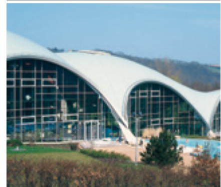
Toskana Thermal Spa, Bad Sulza, Germany
