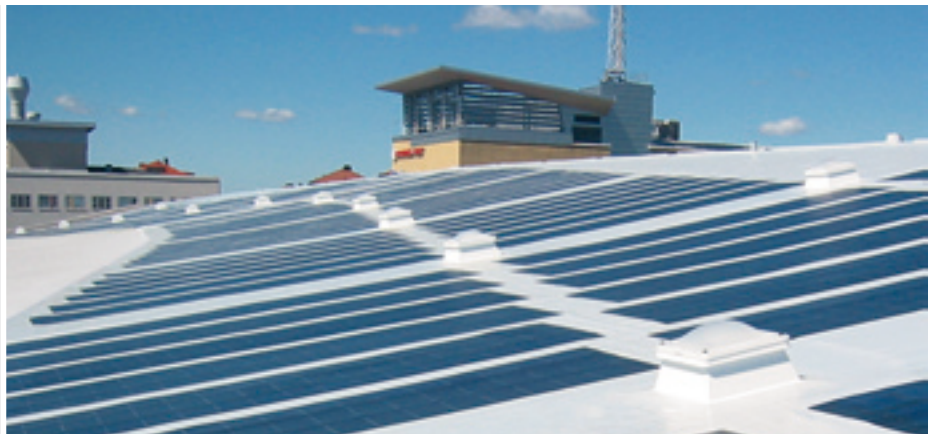
Waterproofing with the world's first roof integrated PV waterproofing membrane EVALON® Solar (Multipurpose Arena HOVET, Stockholm, Sweden)
